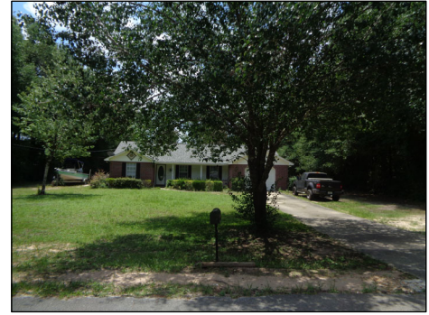
Looking south. Site is behind.
